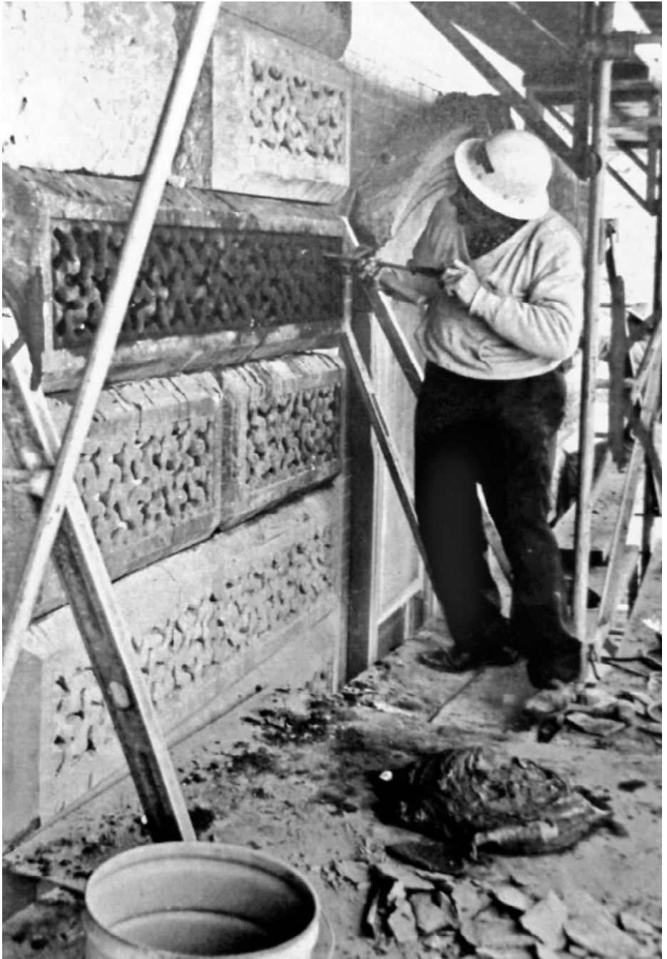
Restoration work on the Renwick Gallery, early 1970s
